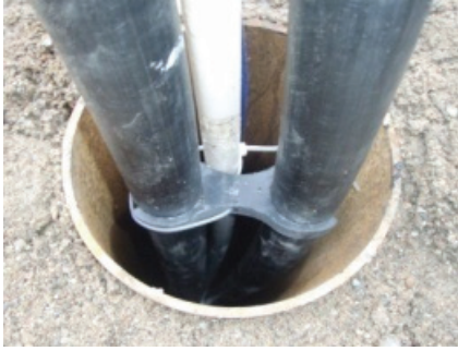
Figure 1. U-pipe BHE with 38 mm spacers
