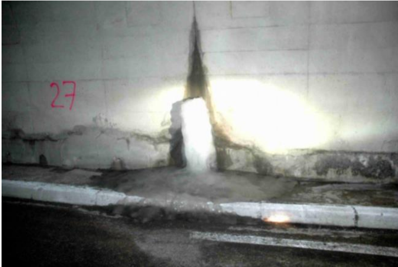
Pack of ice coming from a joint and spreading onto the walkway
